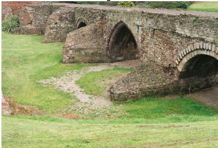
The medieval bridge. KH
