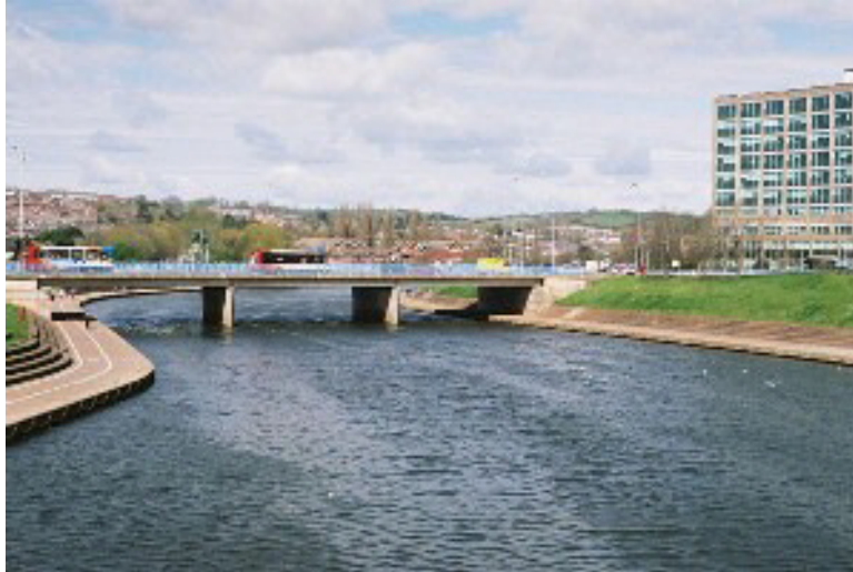
Exe Bridge North KH
