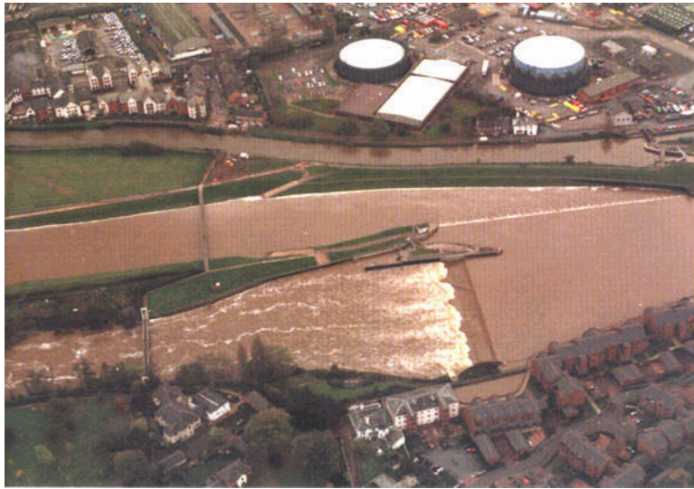
Flood defences protect Exeter, 2000
